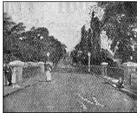
Bridge over mill-stream
